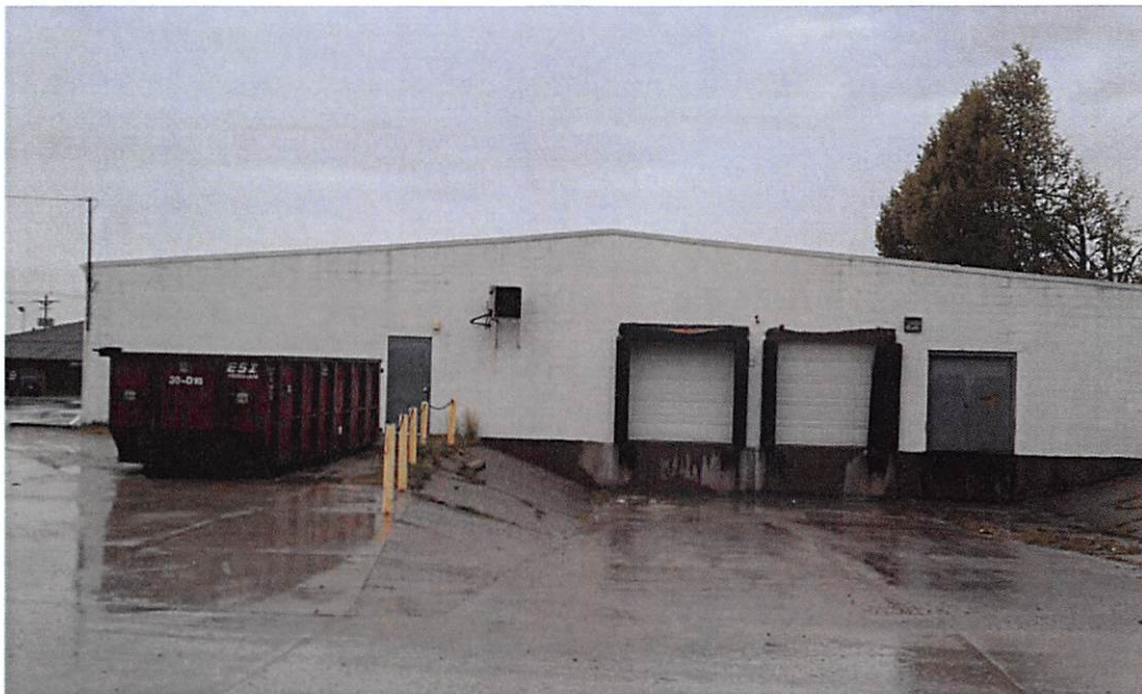
South building elevation-loading well and overhead doors
